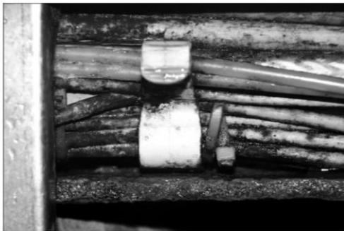
Fig. 2. Biofilm and impurities on the bundles of cable lines underneath the conveyor belt.
