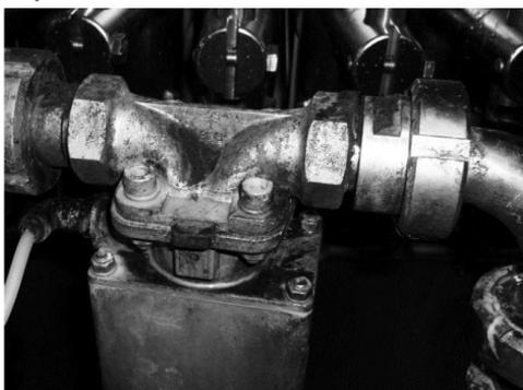
Fig. 5. Biofilm on the surface of pneumatic valve beside the filler.
