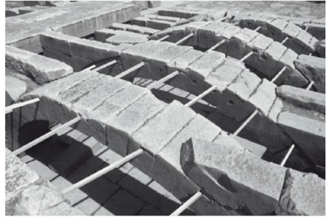
(fig. 26) Moretti's experiment to reconstruct the arch coverings (Photo: Moretti) 139
