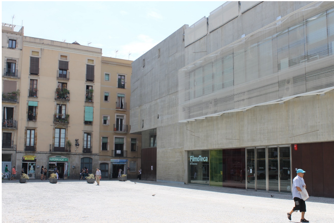
Figure 16. The impressive Filmoteca de Catalunya building (on the right) and a popular residential block in the Illa Robador Area
