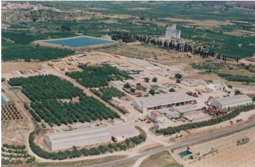
Figure 1. First installations of Ravago Plásticos (Vilallonga, Spain) in the 80s 1
