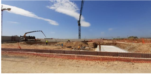
Figure 3.1. Construction of the WWTP.
