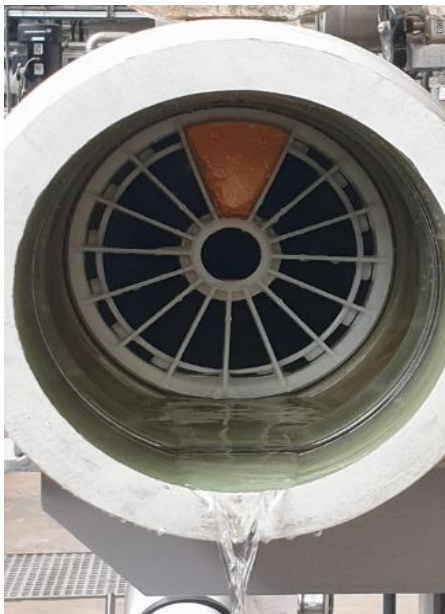
Figure 51 Endcap Stuck inside the Pressure Vessel
