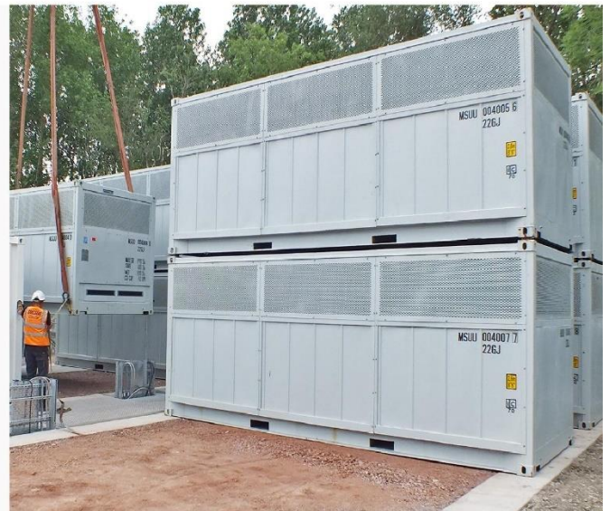
Siting underway. Double-stacked configuration shown
