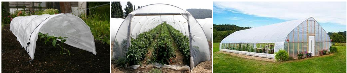
Figure 2.4. Low tunneling, high tunneling and industrial size building greenhouses. (14)
