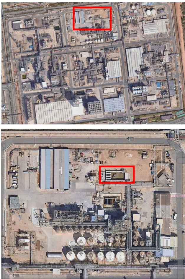
Figure 6.1. Cooling tower location.
