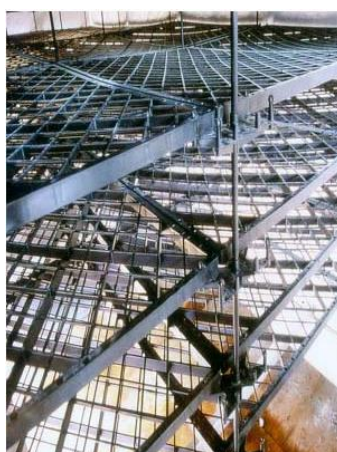
Figure 7.11. Splash-type fill.
