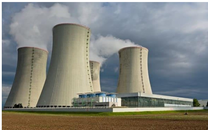
Figure 3.6. Natural draft cooling tower.
