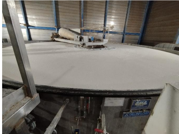
Figure 1.4. Dissolved air flotation system. Own work.
