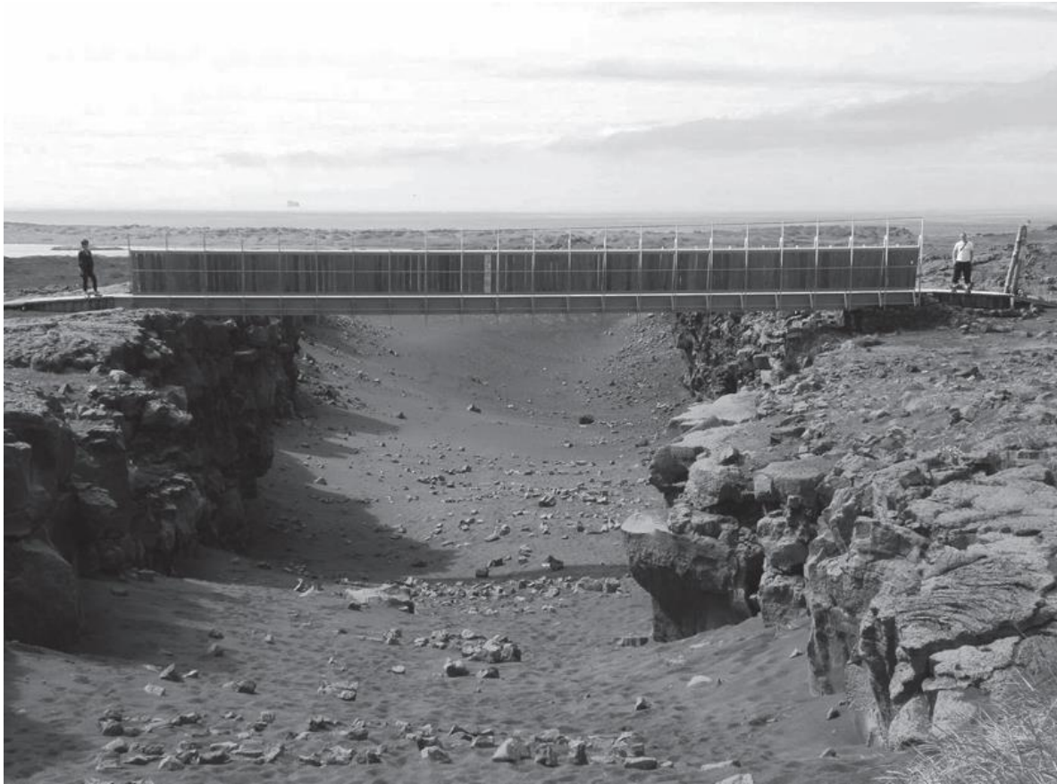
Figure 24. The ‘Bridge Between Two Continents’ Reykjanes peninsula, Iceland. The bridge joins the Eurasian and North American continental tectonic plates. Source: Dowling (2013)
