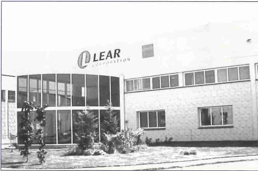
Figure 35. Picture showing the ETC building at Valls-Tarragona (Spain)
