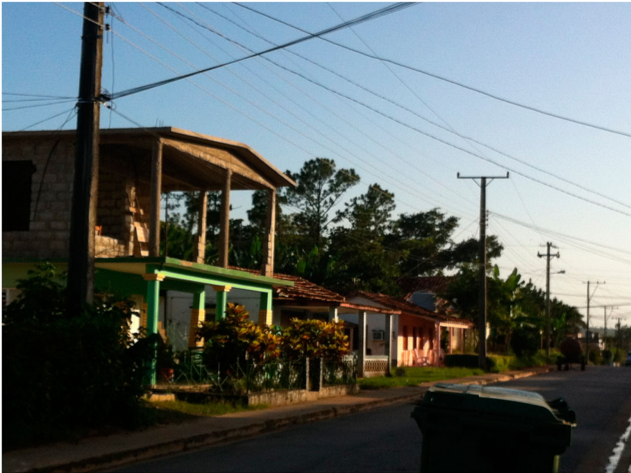
Figure 3. Examples of changes to the heritage in the historical centre of Viñales: an extra floor has been added. Source: authors.
