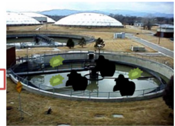
Waste water treatment plant
