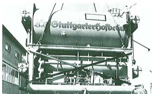
Figure 15: Heat transformer installed in 1986: GEA, nominal capacity \approx 1.4 MW [46]
