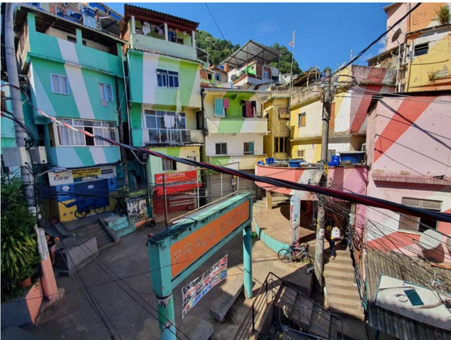
Figure 4. The colorful main square Praça Cantao . Designed and executed by two Dutch artists supported by Coral Tintas in 2012. Bullet holes can be seen on the residences' front walls. Source: Eugenia Altamirano.
