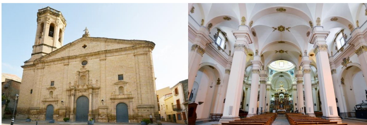
Figure 1. Main façade (exterior) and nave (interior) of the church of Sant Miquel of Batea
