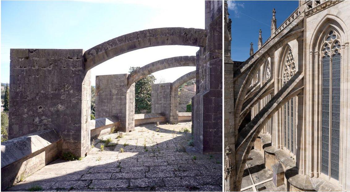
Figure 1. On the left, a picture showing some flying buttresses of Girona Cathedral. On the right, a picture showing some flying buttresses of Narbonne Cathedral. Despite the geographical, historical and architectural influences, there are significant aesthetic differences. Moreover, the flying buttresses in Narbonne, unlike those in Girona, have the function of draining rainwater. (Pictures by the authors).
