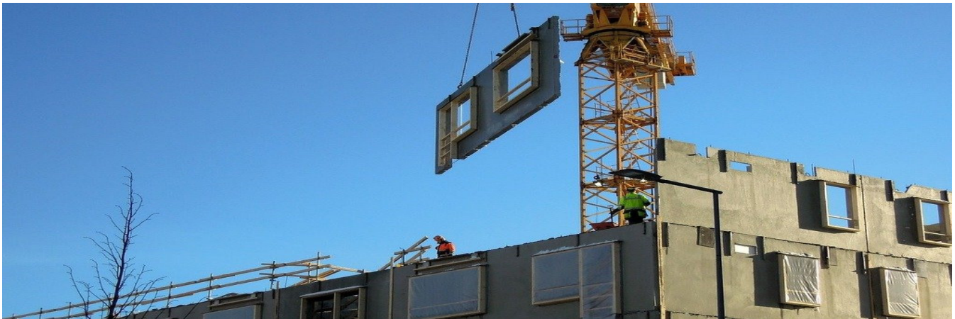
Figure 2. Lifting process of a modular 2D panel used in OSC buildings.
