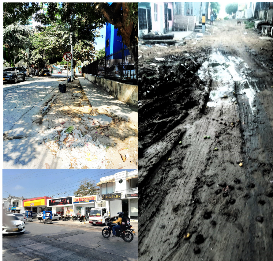
Figure 4. Deteriorated urban roads and sidewalks encroached upon by parked vehicles in Cartagena, Colombia. Source: Zaida Salas-Franco.
